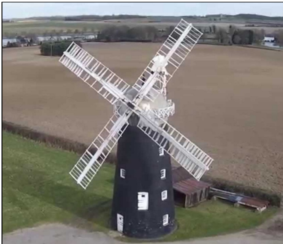
Pakenham Tower Mill
