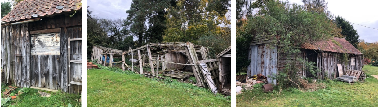
Mill Buildings before demolition
