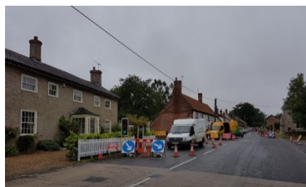
Sewer works in The Street in August
