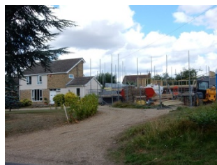
Houses at The Bailey under construction.
