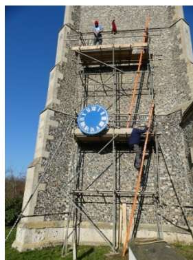
The clock face being hoisted into position in December
